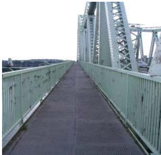
Plate 4.1. Existing narrow footway on the east side of the SJB, that is intended for pedestrians, but is also used by cyclists.
